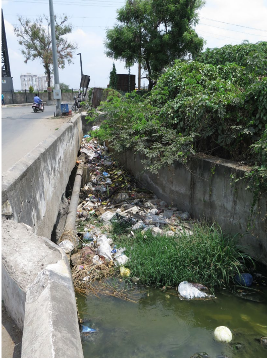
Figure 1: Waste dumping in the outlet of Selvachintamani Lake in April 2022. Source: AQUA-Hub Project Team (Liehr)
