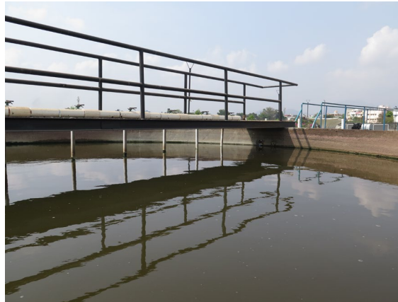
Figure 2: Wastewater Treatment Plant at Selvachintamani Lake in April 2022. Source: AQUA-Hub Project Team (Liehr)
