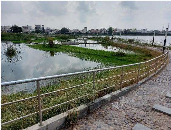
Figure 1: Newly developed walkways at Selvachintamani Lake in April 2022. Source: AQUA-Hub Project Team (Liehr)
