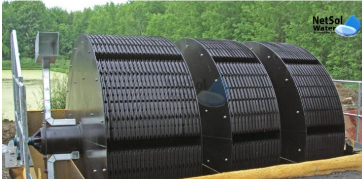
Figure 10: Example of a rotating disc contactor for wastewater treatment (Source: NetSolWater).
