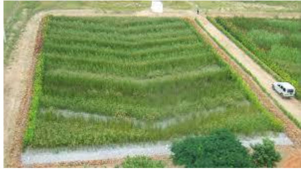
Figure 7: Schematic and example of a constructed wetland for water treatment (Sources: Global Wetland Technology, Biomatrix)
